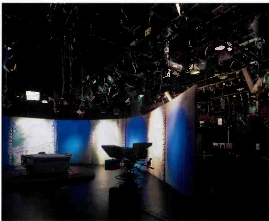
KQED's Studio A, a 4,000-square-foot studio for large productions, features a unique bilevel air distribution system and a fully motorized lighting batten system.
